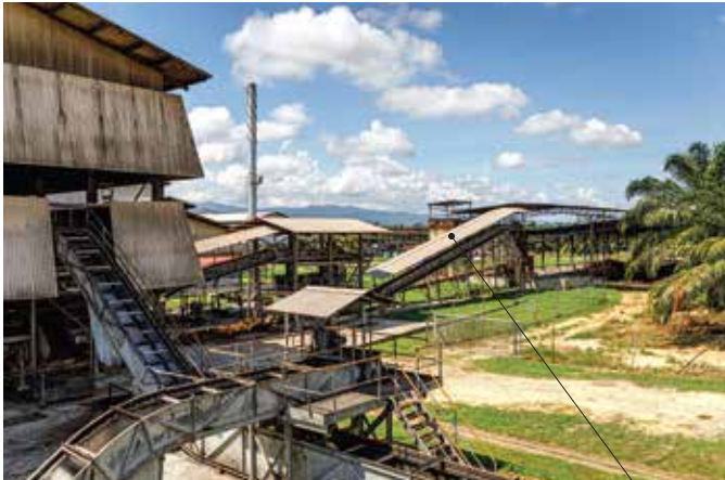
Palm oil conveyor and elevator
